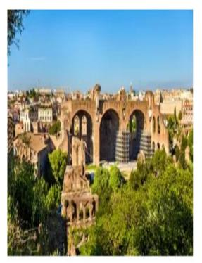
with a span of 26 metres. All of these buildings contained stone columns, but they were purely ornamental and could have been removed at will. The brick-faced concrete walls were left exposed on the exteriors, but the interiors were lavishly decorated with a veneer of thin slabs of coloured stone held in place by metal fasteners that engaged slots cut in the edges of the slabs, a technique still used in the 20th century
